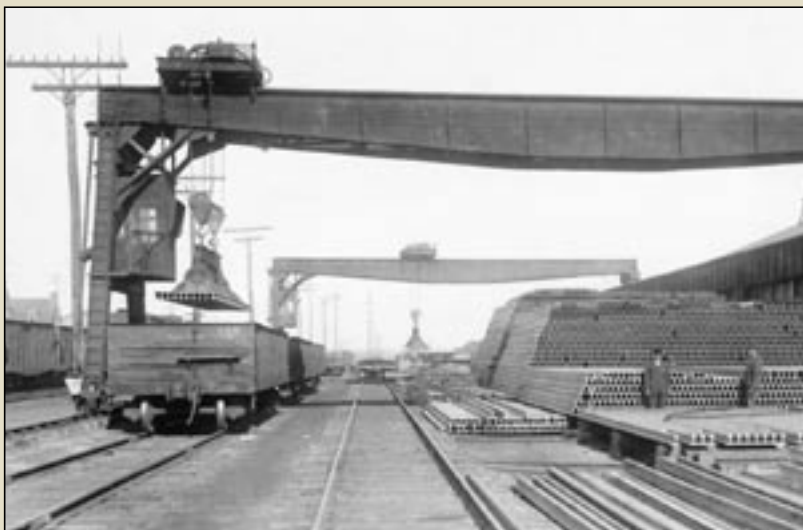
Finished rails are stacked into gondola cars by an electromagnet traveling crane.
