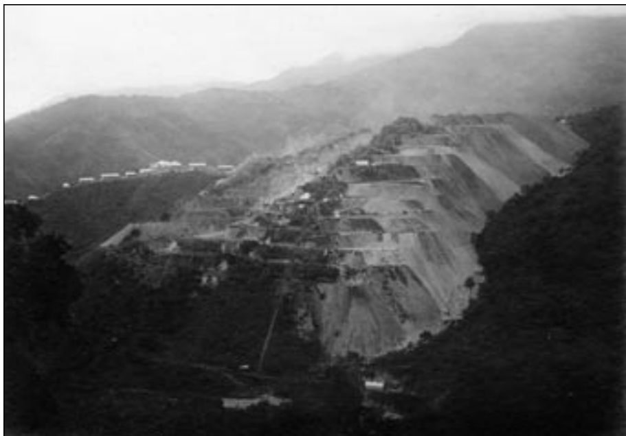
Lola Hill took on the look of a giant corkscrew as it was stripped of its ore. Marion steam shovels worked on the different shelves, removing ore that was blasted out of the rock face by black powder and dynamite. Note the miners' barracks in the distance.
