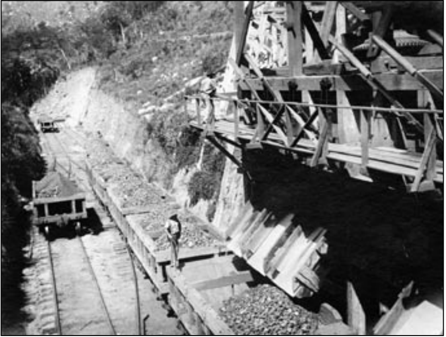
Ore is loaded into railway cars at the bottom of Lola Hill for the short ride (five miles) to the Daiquiri pier and the long ocean journey (1,300 miles) to Sparrows Point.
